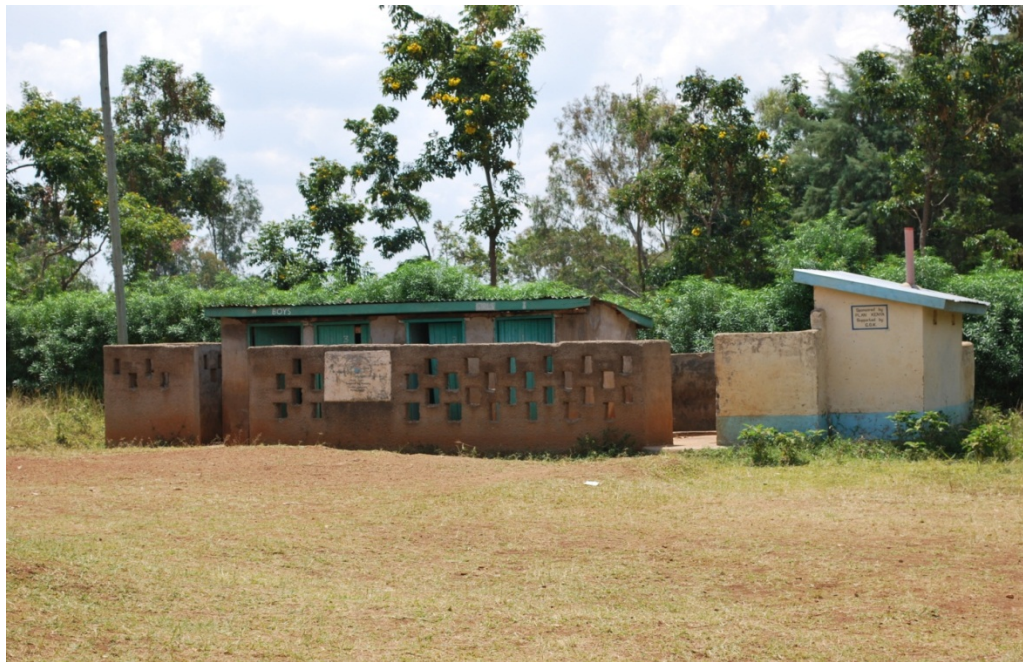
Figure 12: Pit latrines at Nduru-Kadero school
